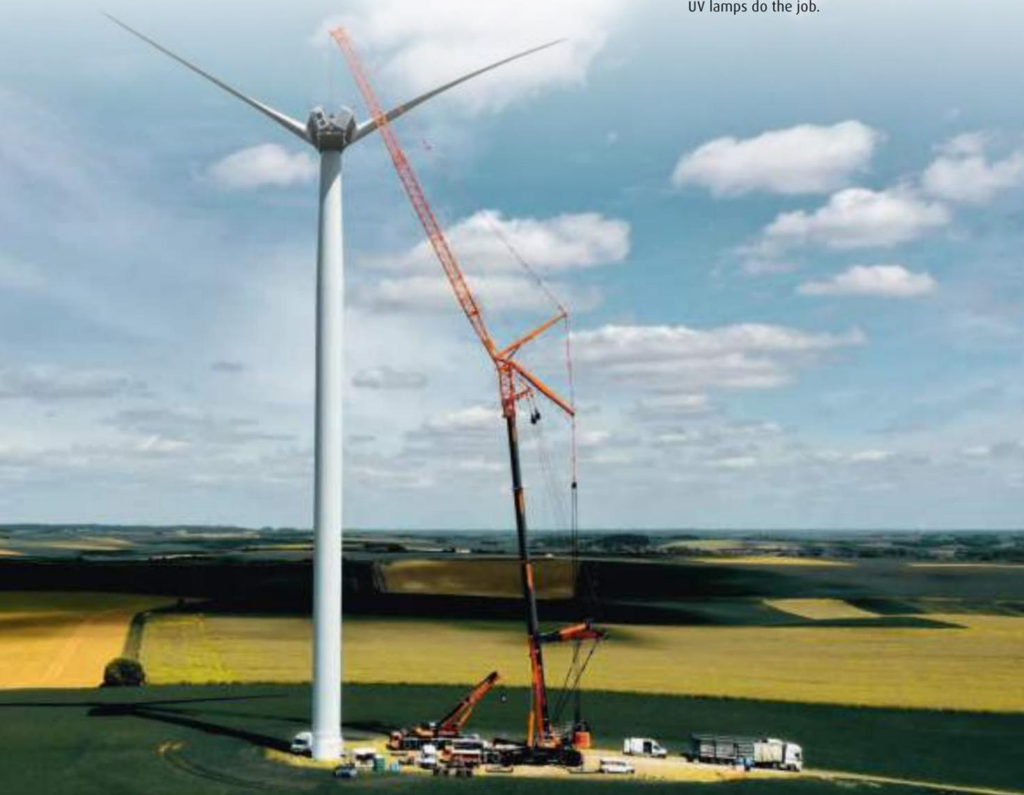
**Main component replacements:** the ENERTRAG Service team replaces main and yaw gears, rotor bearings and generators.
