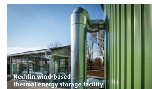
Nechlin wind-based thermal energy storage facility
