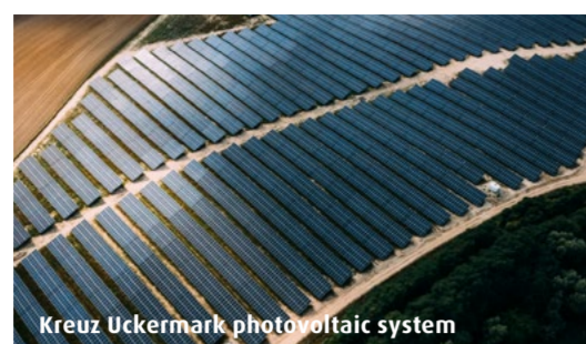
Kreuz Uckermark photovoltaic system
